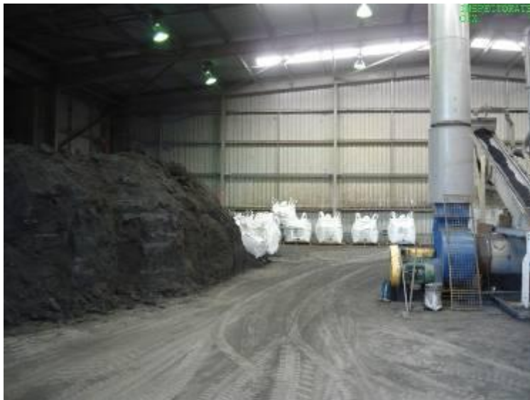
Bags stored close to stockpile in storage shed
