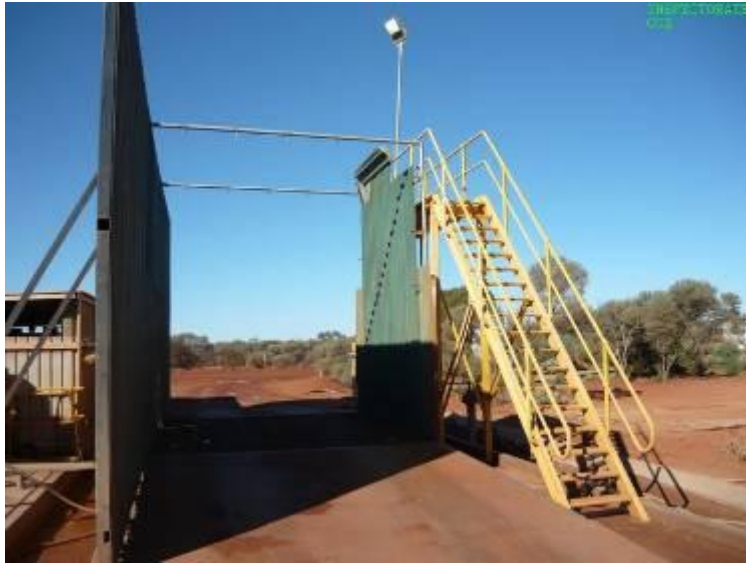
Truck Wash Facility
