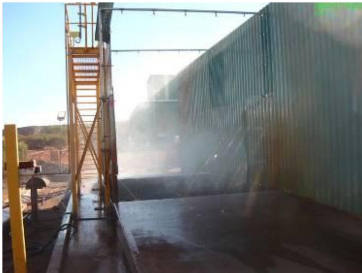
Truck Wash Facility
